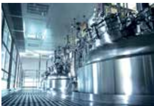
Tank and silo weighing
