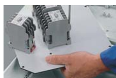
Device installation on mounting plates
