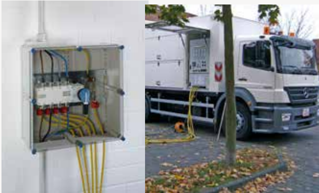
Changeover switch boxes (I-0-II) switch safely to substitute power sources
