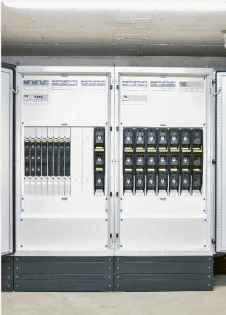
Outdoor installation of an Mi distribution board in front of a university building in India
