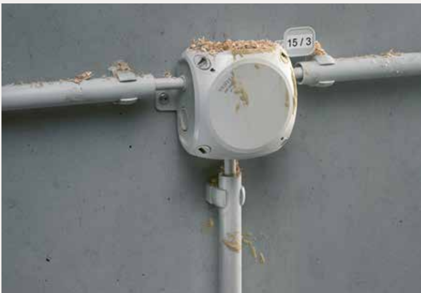
The HENSEL cable junction box is dustproof (IP 66).
