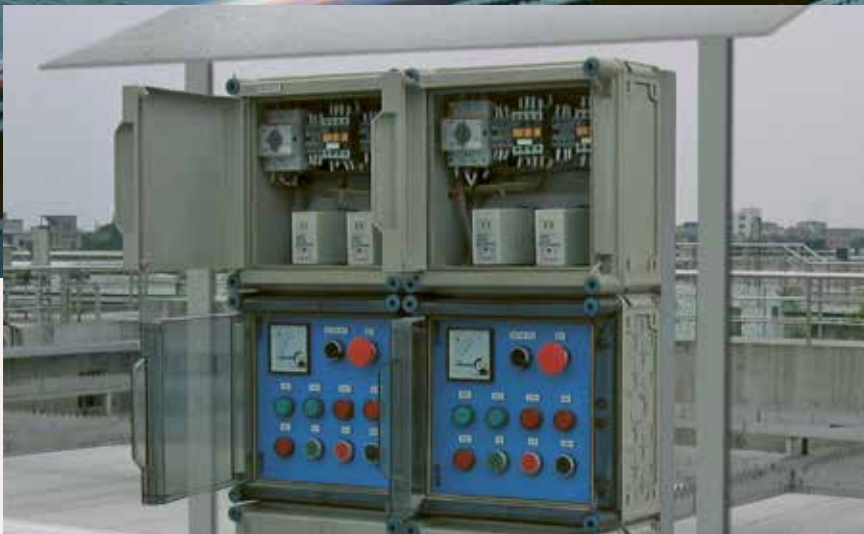
Water treatment and sewage plants in China
