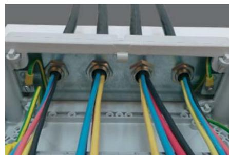
Cable entry for armoured cables via metal glands
