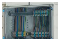
Terminals for incoming/outgoing cables under accessories
