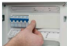
Blanking strips for unused DIN rail openings
